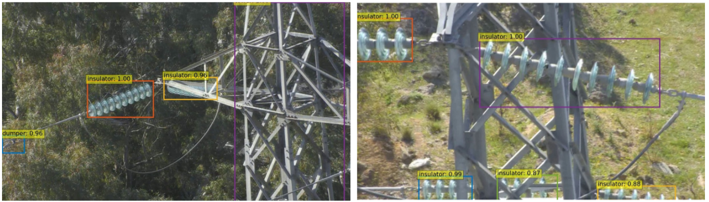
Fig. 1. Examples of our powerline inspection dataset and elements detected by DETR.
